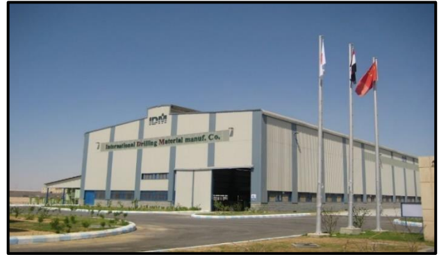
IDM CASING&TUBING AIN SOKHAN, EGYPT
