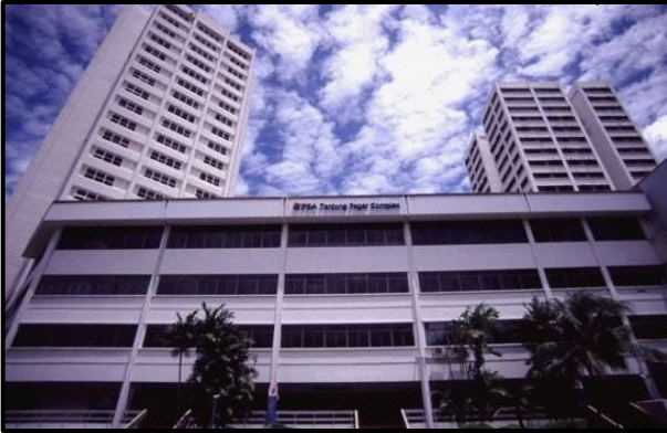
TANJONG PAGAR COMPLEX PSA BUILDING, SINGAPORE
