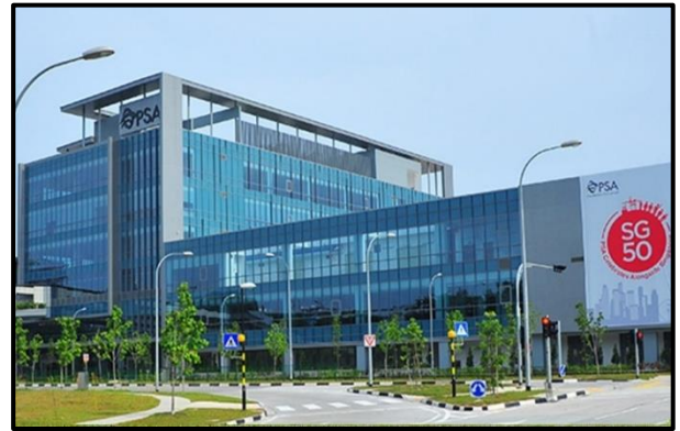
PASIR PANJANG TERMINAL 1 PSA BUILDING, SINGAPORE
